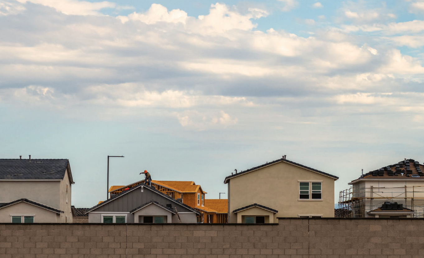
■ A roofer works on a home in a housing development in Buckeye, Arizona, in September.
