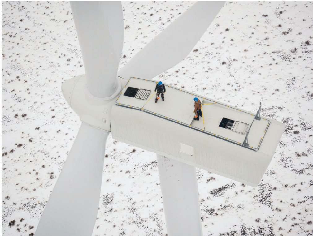
Workers at Wild Horse Wind Farm in central Washington. Kyle Johnson
