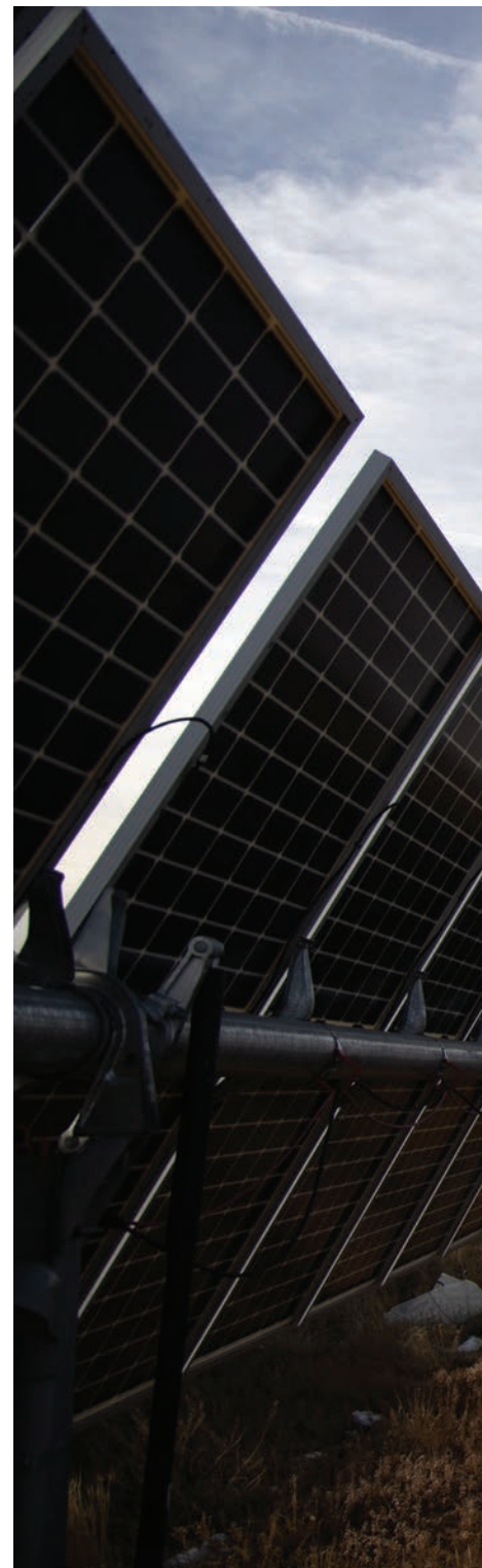
Kit Carson's largest solar array, near Taos, New Mexico. Renewable energy now provides 100% of the year-round daytime electrical needs of the energy co-op's more than 30,000 members.
