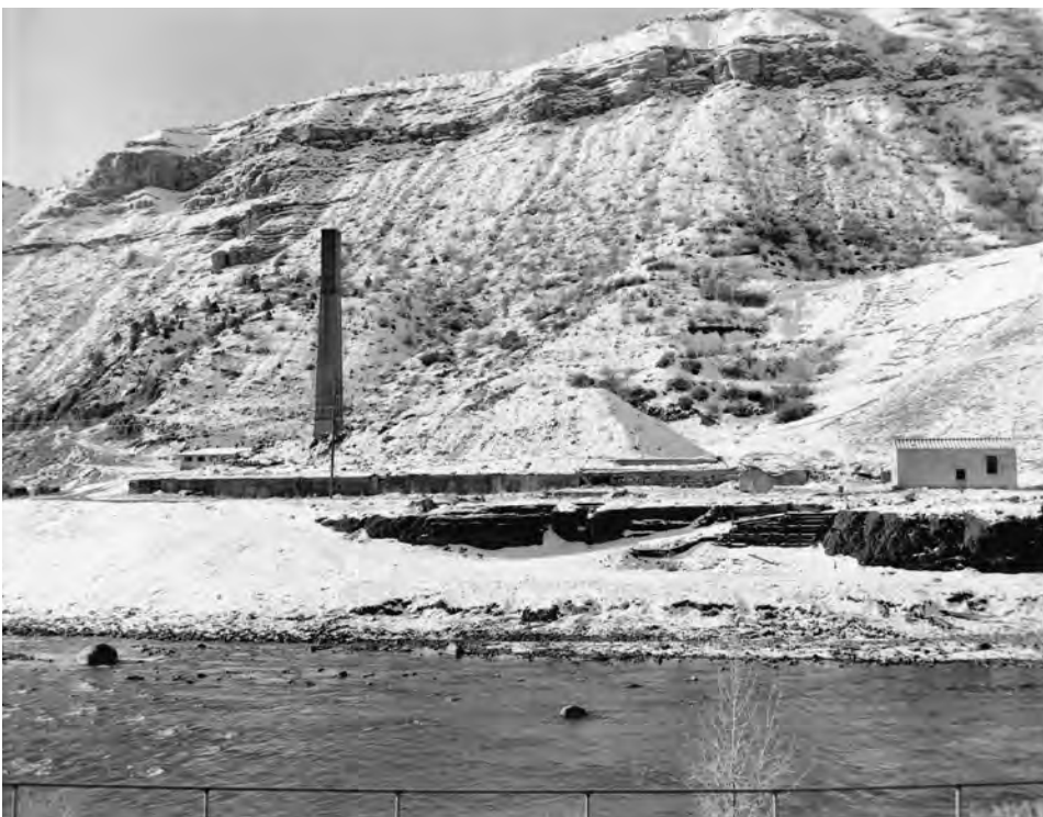
Navajo miners operate a mucking machine at the Rico Mine in 1953, where pyrite was extracted to use in the manufacture of sulfuric acid for uranium processing, top. Above, the smelter, stack and tailings pile along the Animas River, where uranium was processed.
