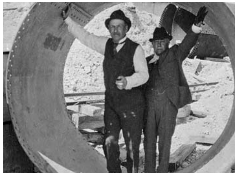
William Mulholland and Commissioner Del Valle in an 80-inch pipe at Power Plant 1 construction in 1916. LOS ANGELES DEPARTMENT OF WATER AND POWER
