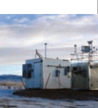
A Wyoming DEQ-Air Quality Division monitoring station used to study ozone formation in the Upper Green River Basin. BLM
