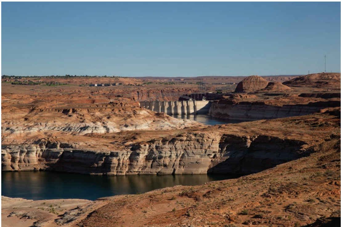
The water level at Lake Powell continues to drop and could soon threaten the electricity-generating turbines of Glen Canyon Dam, seen in the distance. Luna Anna Archey / HCN
