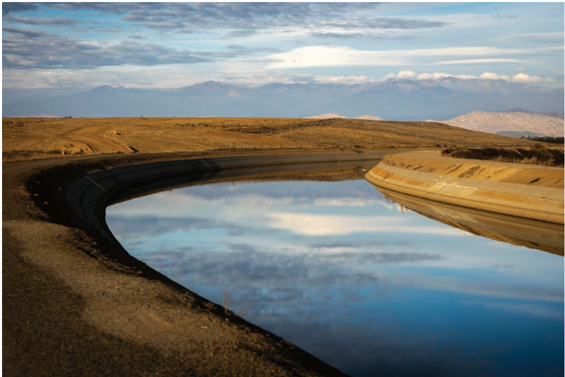
The Friant-Kern Canal as it passes through Terra Bella, California, with the peaks of the Sierra Nevada in the background. Subsidence is causing water flow issues in and around Terra Bella, but is hard to see, as it spans a 30-mile stretch of the canal. Martin do Nascimento / HCN
