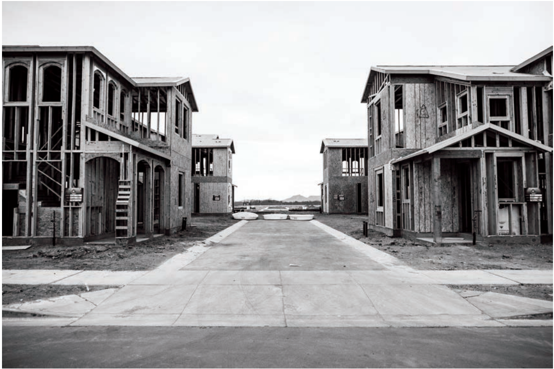
With a waiting list for new homes, construction can't keep up with demand in the Cadence subdivision in Mesa, Arizona. Roberto (Bear) Guerra / HCN
