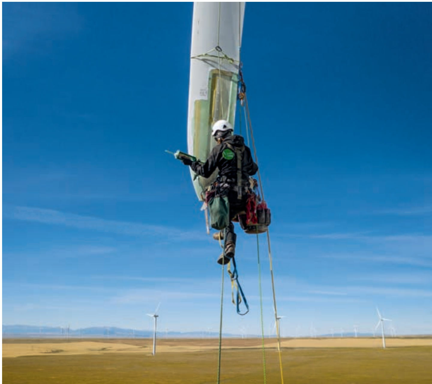
A Rope Partnertechician services a wind turbine blade in the big sky above Judith Gap, Montana. BLAKE GORDON © 2020 Patagonia, Inc.
