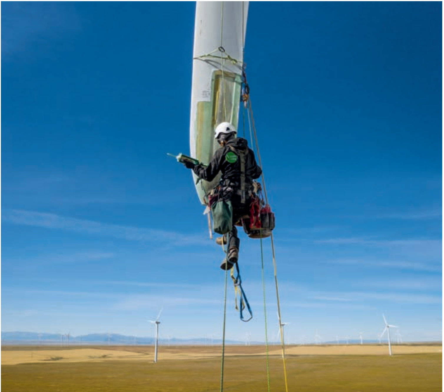
A Rope Partner technician services a wind turbine blade in the big sky above Judith Gap, Montana. BLAKE GORDON © 2020 Patagonia, Inc.
