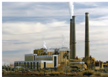
A coal-fired power plant in Hunter, Utah. "ARBYREED," CC VIA FLICKR
