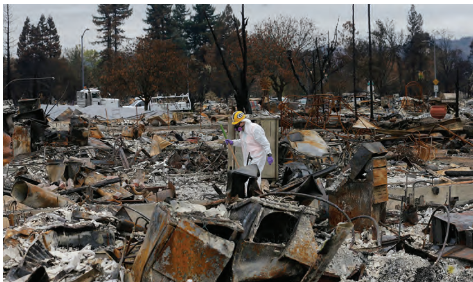
Work crews clean up Santa Rosa, California, after the Tubbs Fire in 2017. JEFF CHIU/AP IMAGES FILE
