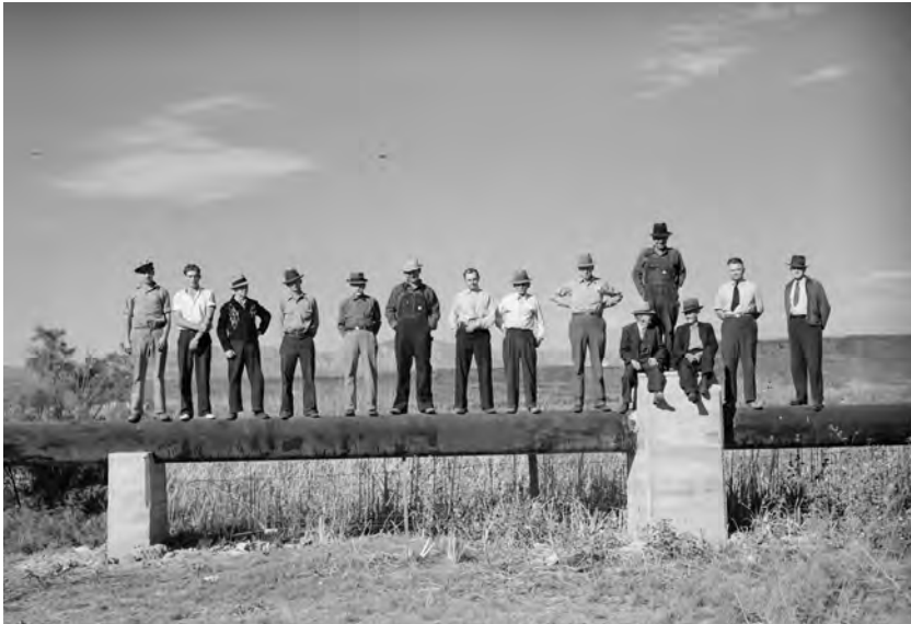
Farm Security Administration members pose on a cooperative pipeline used for irrigation in St. George in 1940. LIBRARY OF CONGRESS
