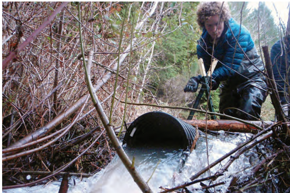
Jakob Shockey of Beaver State Wildlife Solutions installs a pond leveler in Little Canyon Creek, on Susan Sherosick's property outside Sutherlin, Oregon.
