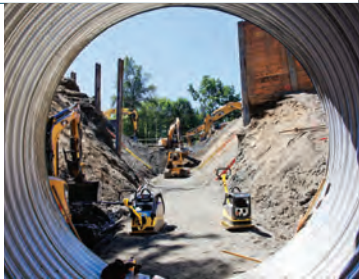
A fish-friendly culvert is built under a state highway near Seattle.
