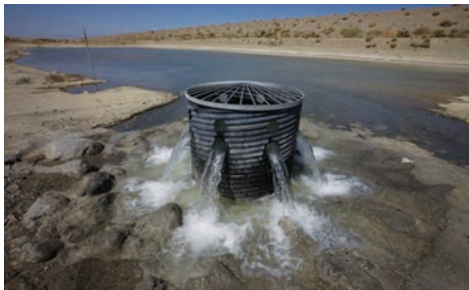
A groundwater recharge facility for the Coachella Valley adds water imported from the Colorado River to the valley's main aquifer and prevents the land from sinking and damaging the surrounding infrastructure. BRENT STIRTON/GETTY IMAGES
