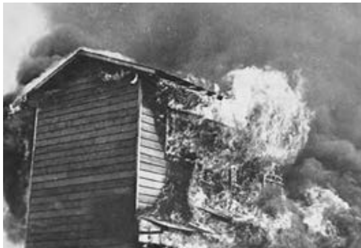
A model German apartment building goes up in flames during a test of the M-69 incendiary bomb in the 1940s at Dugway Proving Ground, in Utah.
