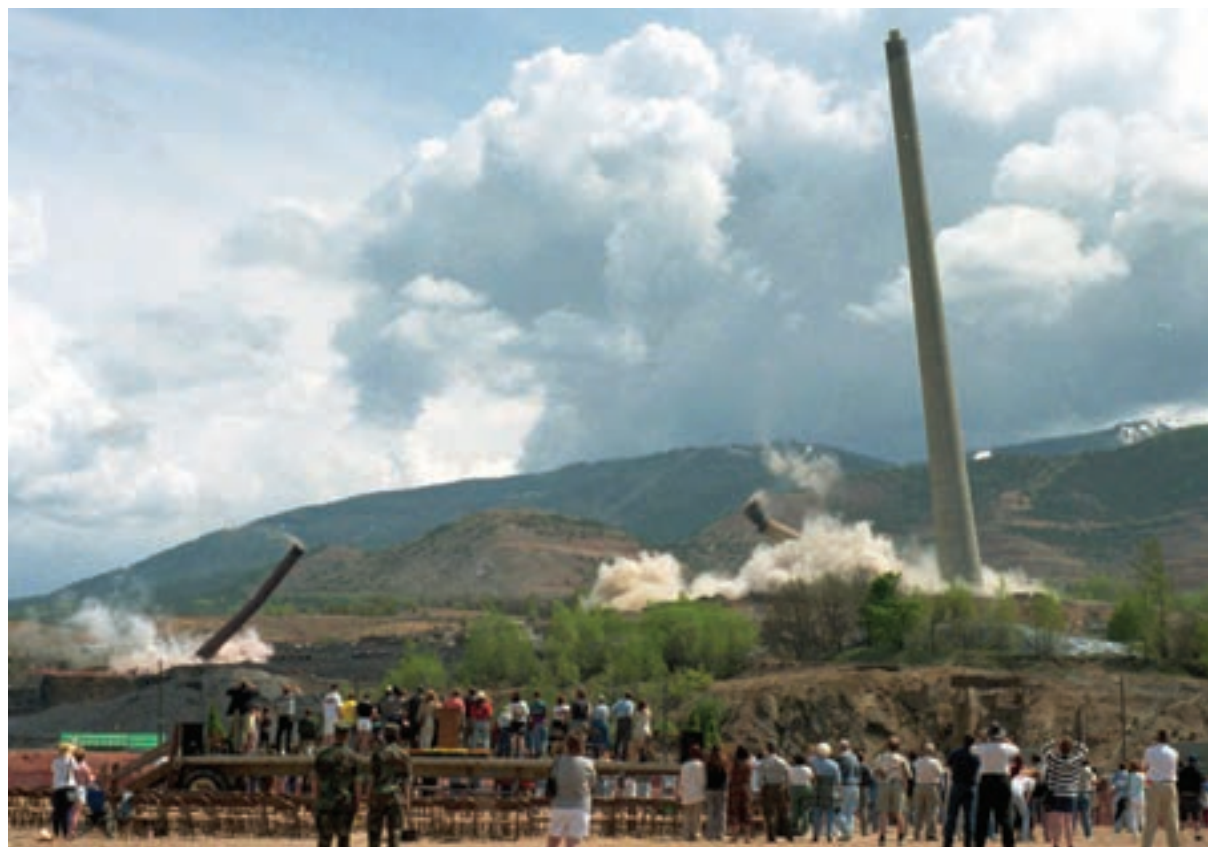
Spectators watch as three of four lead smelting smokestacks are demolished at the Bunker Hill Superfund Site near Kellogg, Idaho, in 1996. RON SWORDS/AP PHOTO
