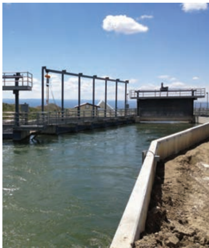
The South Canal Hydroelectric Project is one of Delta-Montrose Electric Association's local renewable energy projects, and is the largest local member hydroelectric project within the Tri-State membership. DMEA
