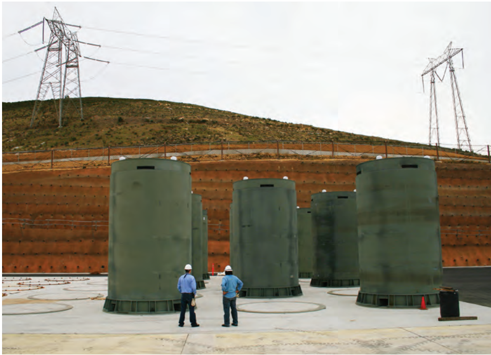
Spent nuclear fuel is stored in steel cylinders called dry casks at the Diablo Canyon nuclear power plant. There's still no long-term disposal method for the waste. NUCLEAR REGULATORY COMMISSION
