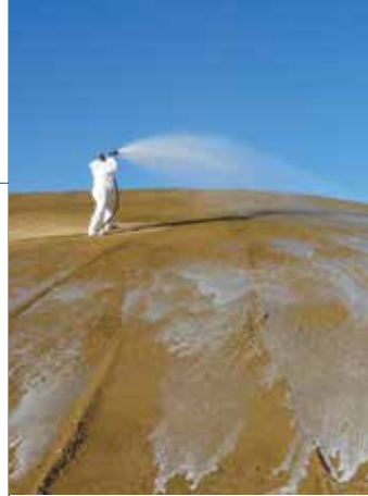
Soil tackifier solution is applied to the dirt around an abandoned uranium mine in Thoreau, New Mexico, to reduce erosion on the contaminated site. ENVIRONMENTAL PROTECTION AGENCY
