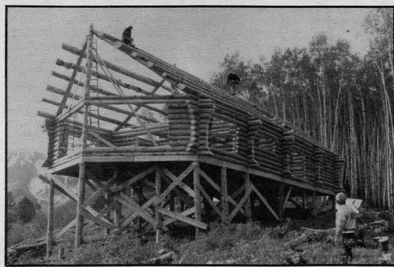
Photo furnished by Tom Chapman showing construction work in June
