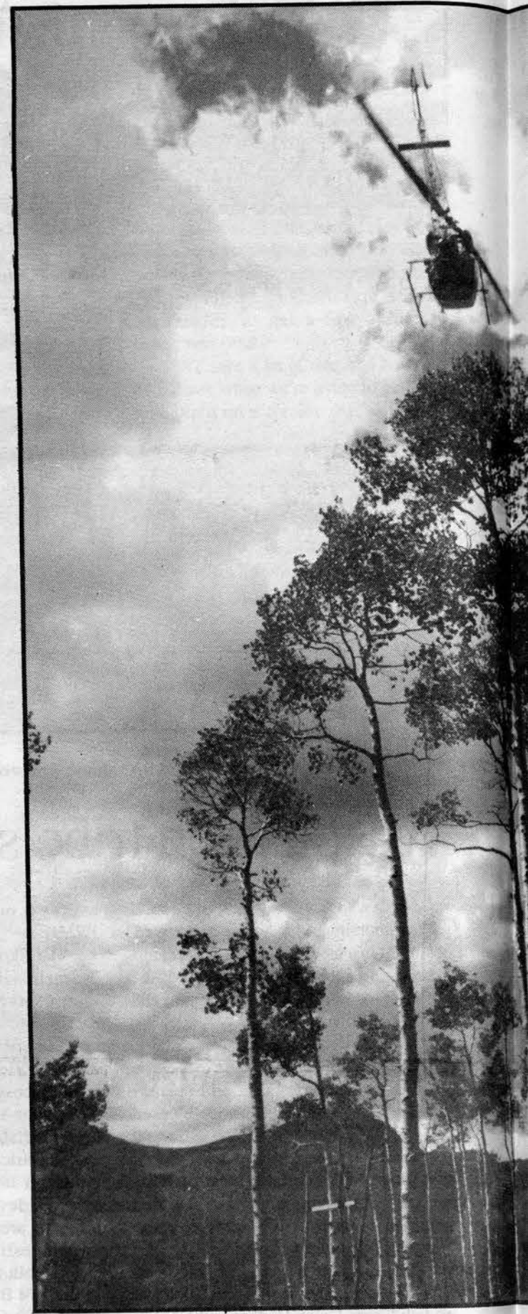
A helicopter lowers building materials into the Tom Chapman
