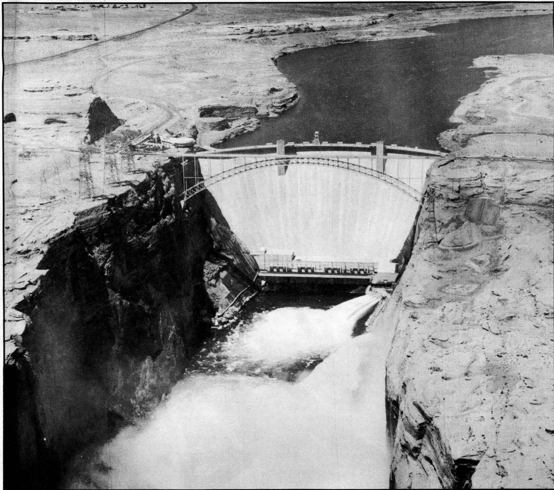
The Glen Canyon Dam and its spillway
