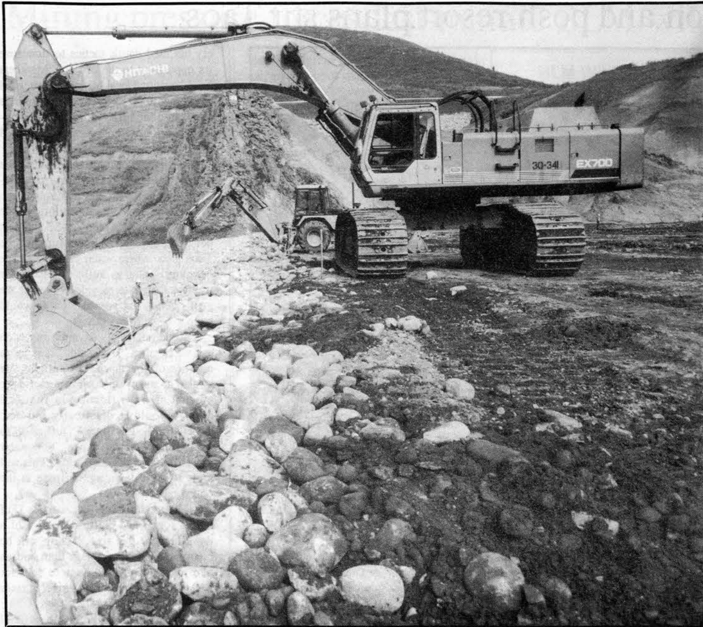
A giant backhoe places material at the Jordanelle Dam site
