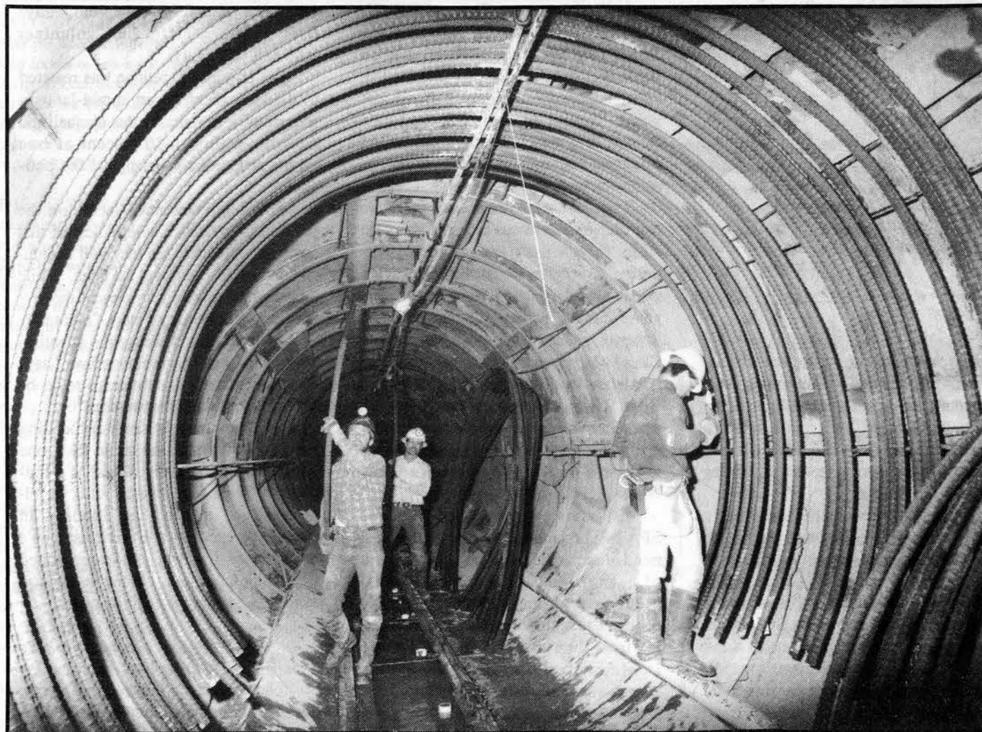
Workers install hoop bar in the Syar Tunnel
