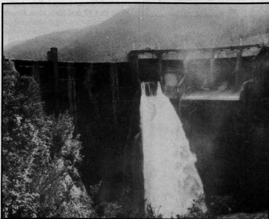
Washington's Glines Canyon Dam on the Elwha River
