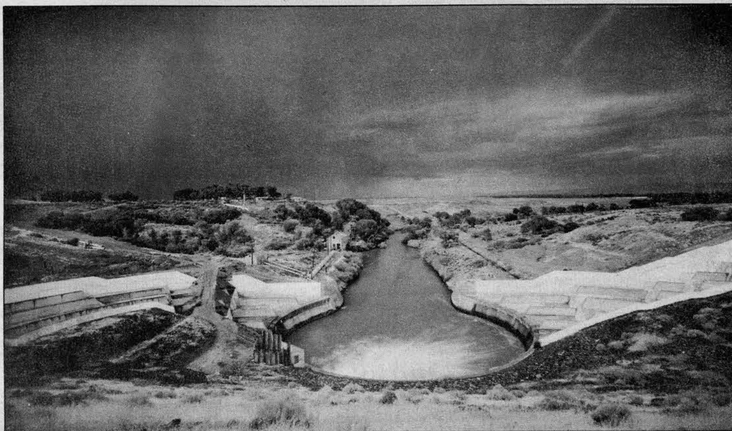
Nevada: The spillway at Lahontan Reservoir near Fallon. Once the Carson River flowed into the Carson Sink creating 800,000 acres of wetlands. These wetlands were a major resting ground for migratory waterfowl and shorebirds. Now the Carson River water is impounded in the Lahontan Reservoir, where it is supplemented with irrigation water highly contaminated with minerals. Only about 26,000 acres of wetlands remain, and some biologists predict that without supplies of fresh water the wetlands will shrink to 10,000 acres, disappearing altogether in dry years. 1984.
