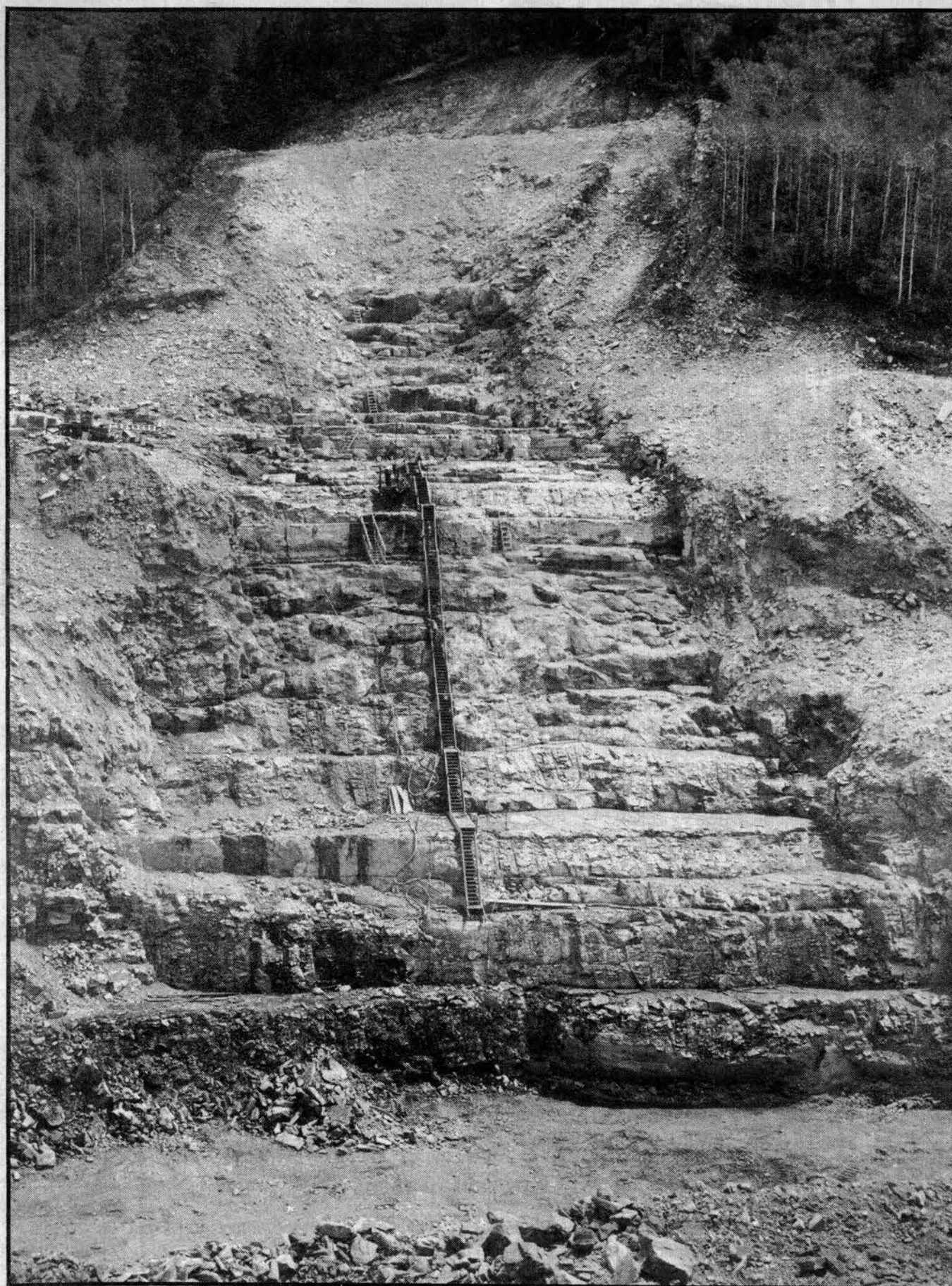
Construction at Exxon's Colony Shale Oil project in Colorado, 1981
