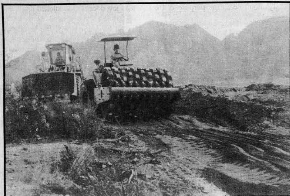
Bulldozing land in Arizona for new homes
