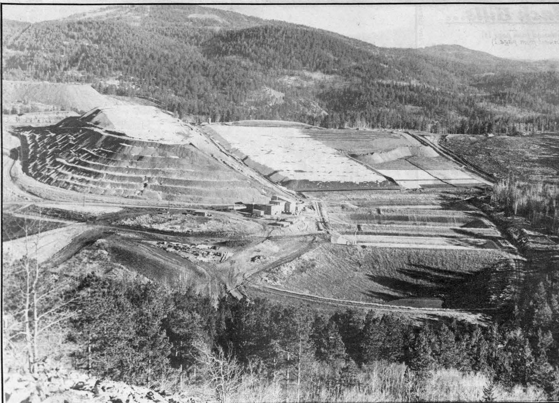
Part of Wharf's open pit mine in the Black Hills
