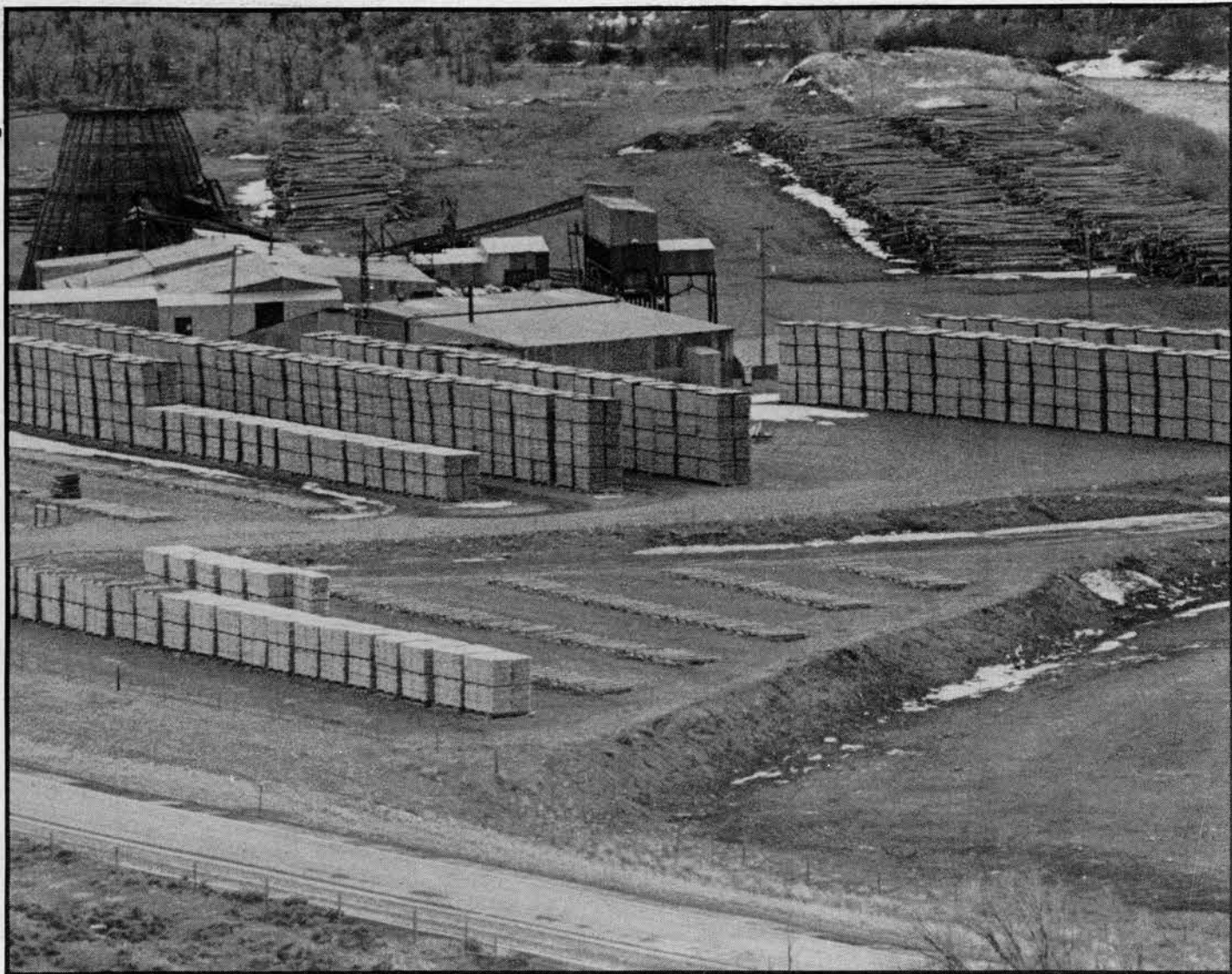
Louisiana-Pacific's stud plant in Dubois, Wyoming
