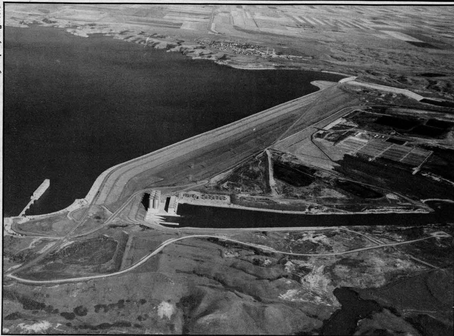
Garrison Dam and Lake Sakakawea, North Dakota
