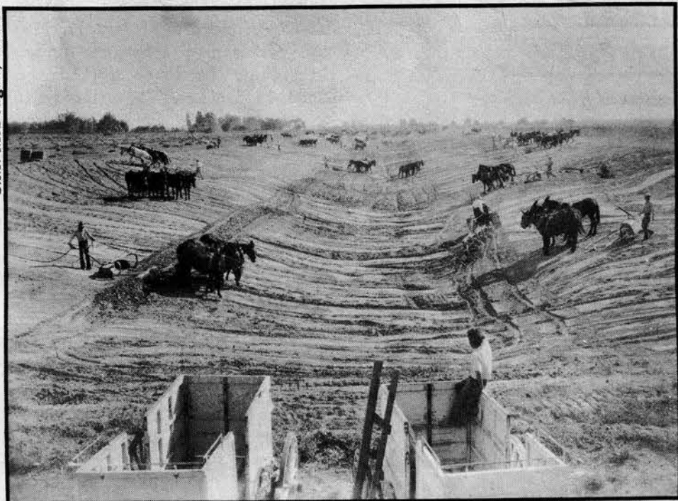
Construction of the All-American Canal, 1935
