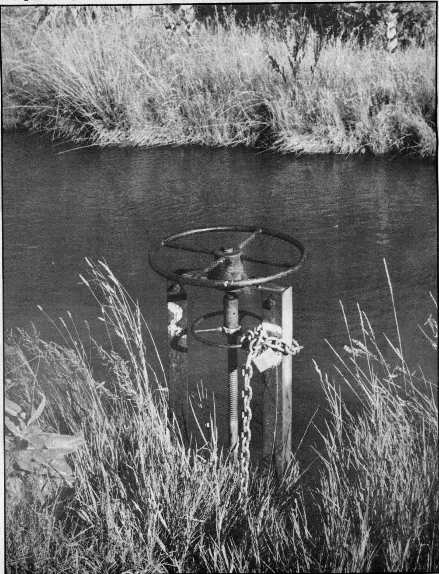
Irrigation canal and outlet gate
