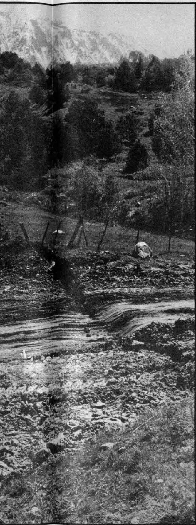
This fracture marks the northern edge of the main slide lobe, about one-fourth mile above the lower end of the slide.
