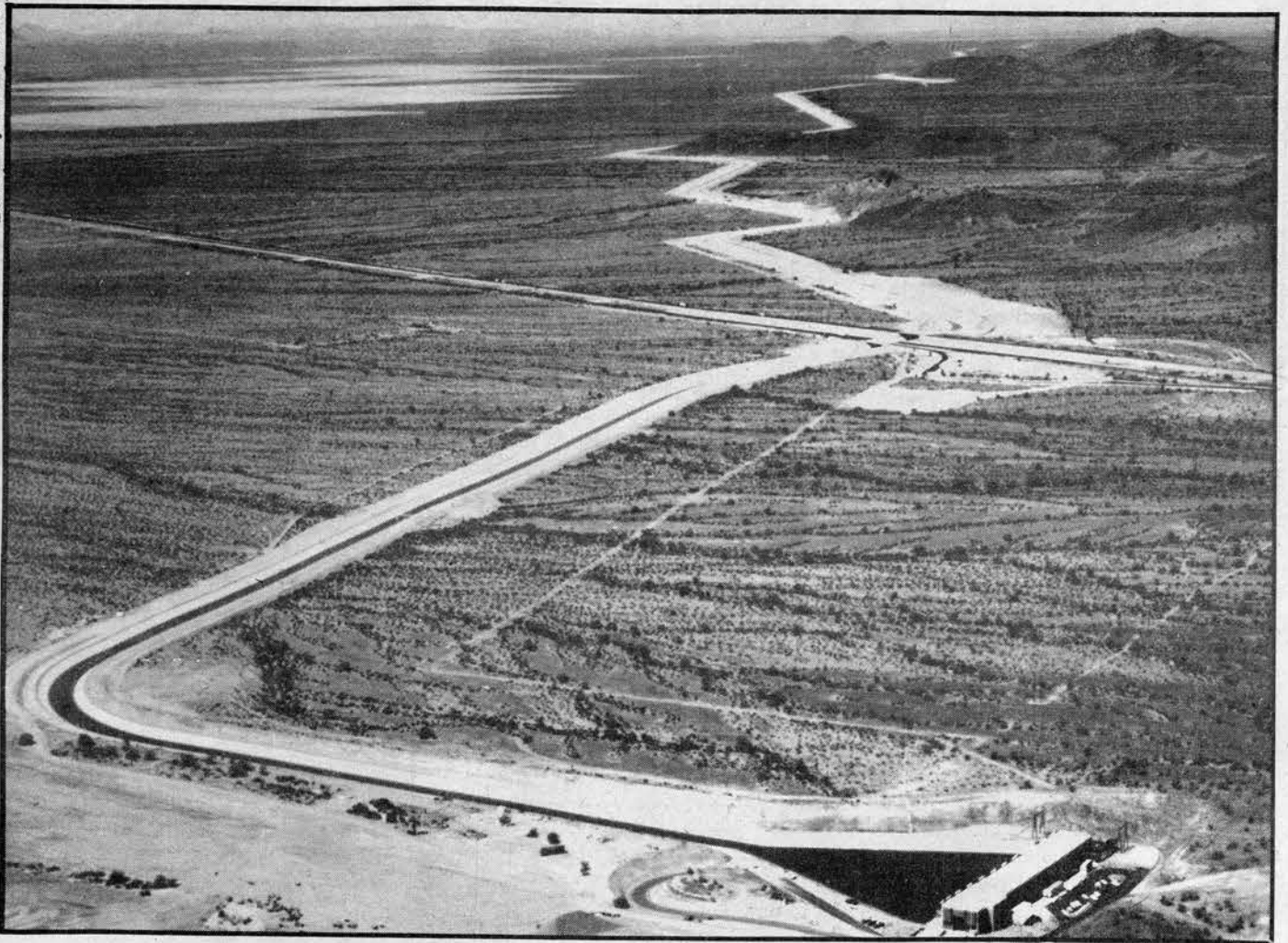
The Little Harquabala Pumping Plant, 30 miles west of the Harquabala Valley Irrigation District turnout
