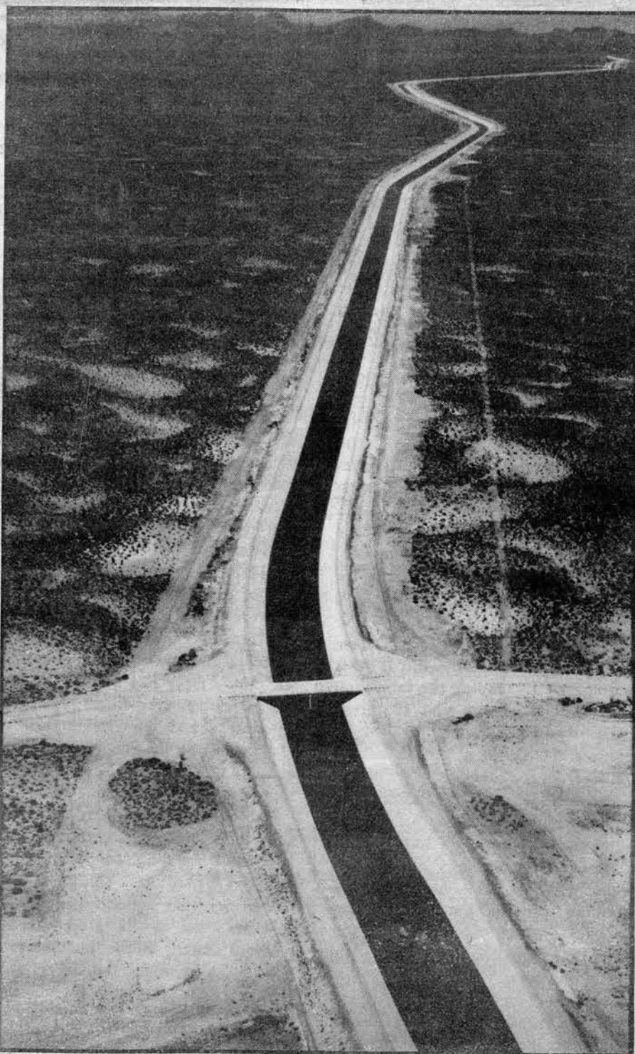
CAP's Granite Reef Aqueduct
