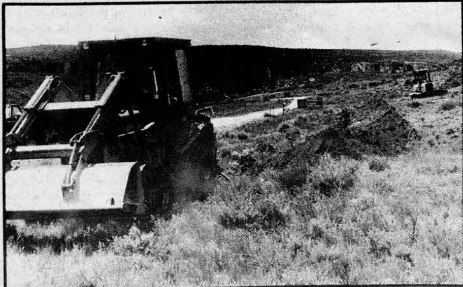
Richard Mott's bulldozers at Black Canyon, June 14
