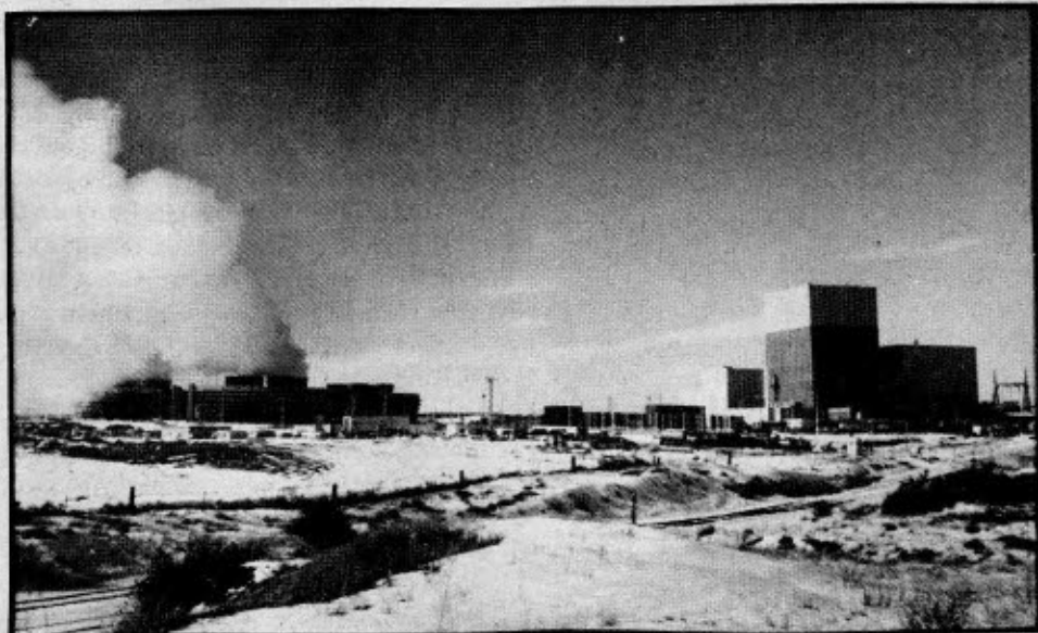
Nuclear power plant #2 with water cooling towers on the left
