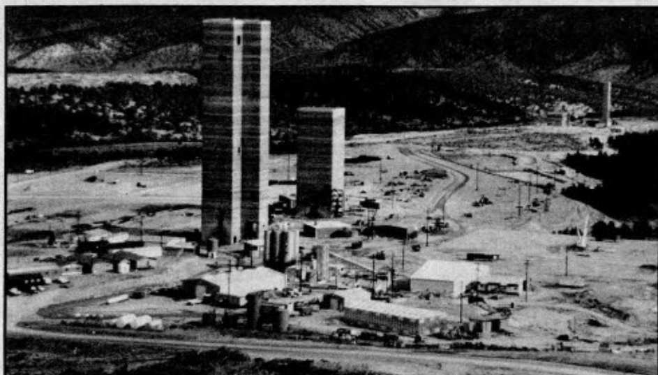
Cathedral Bluffs Shale Oil Plant
