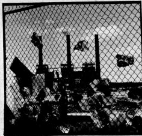
Bridger Power Plant
