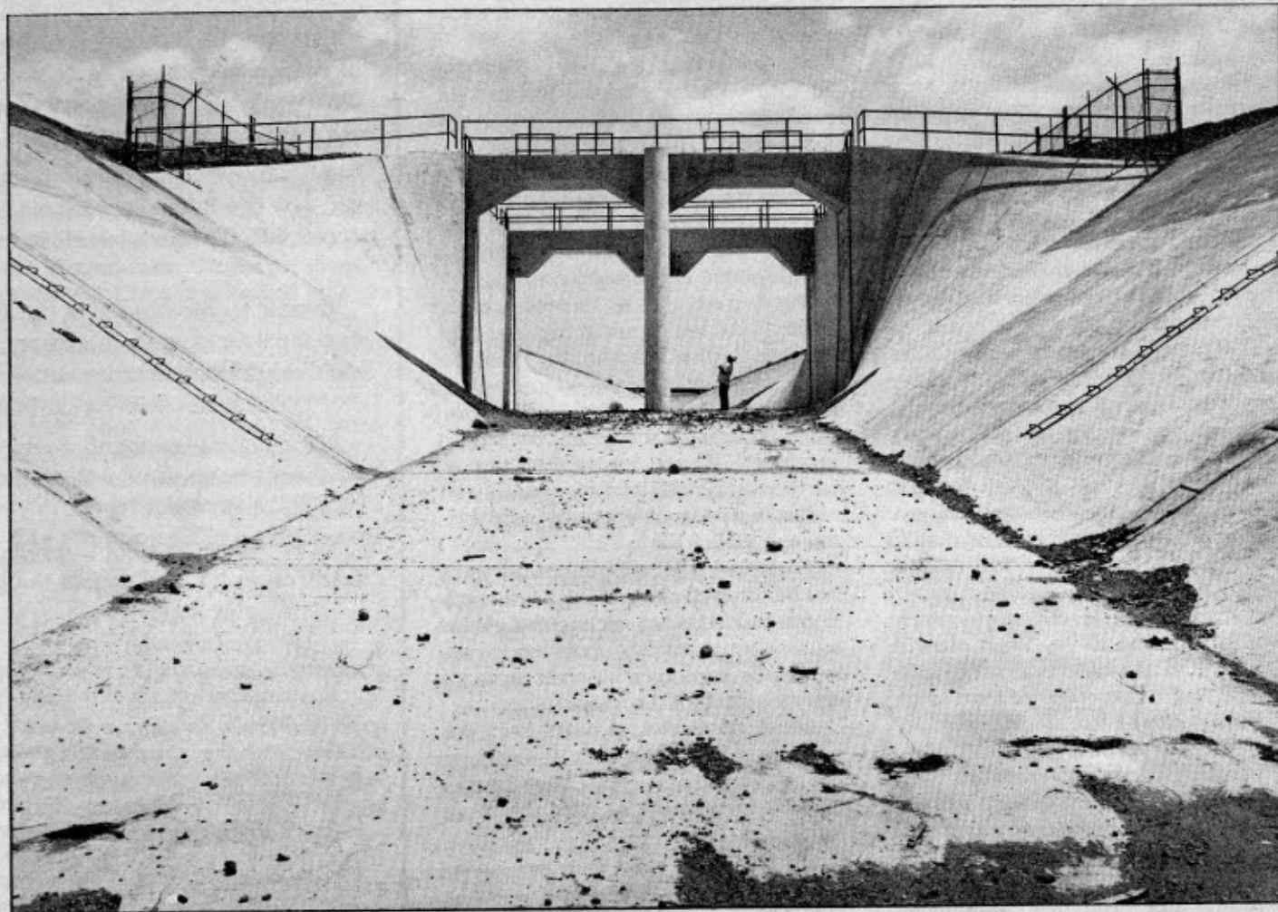
Bureau of Reclamation
