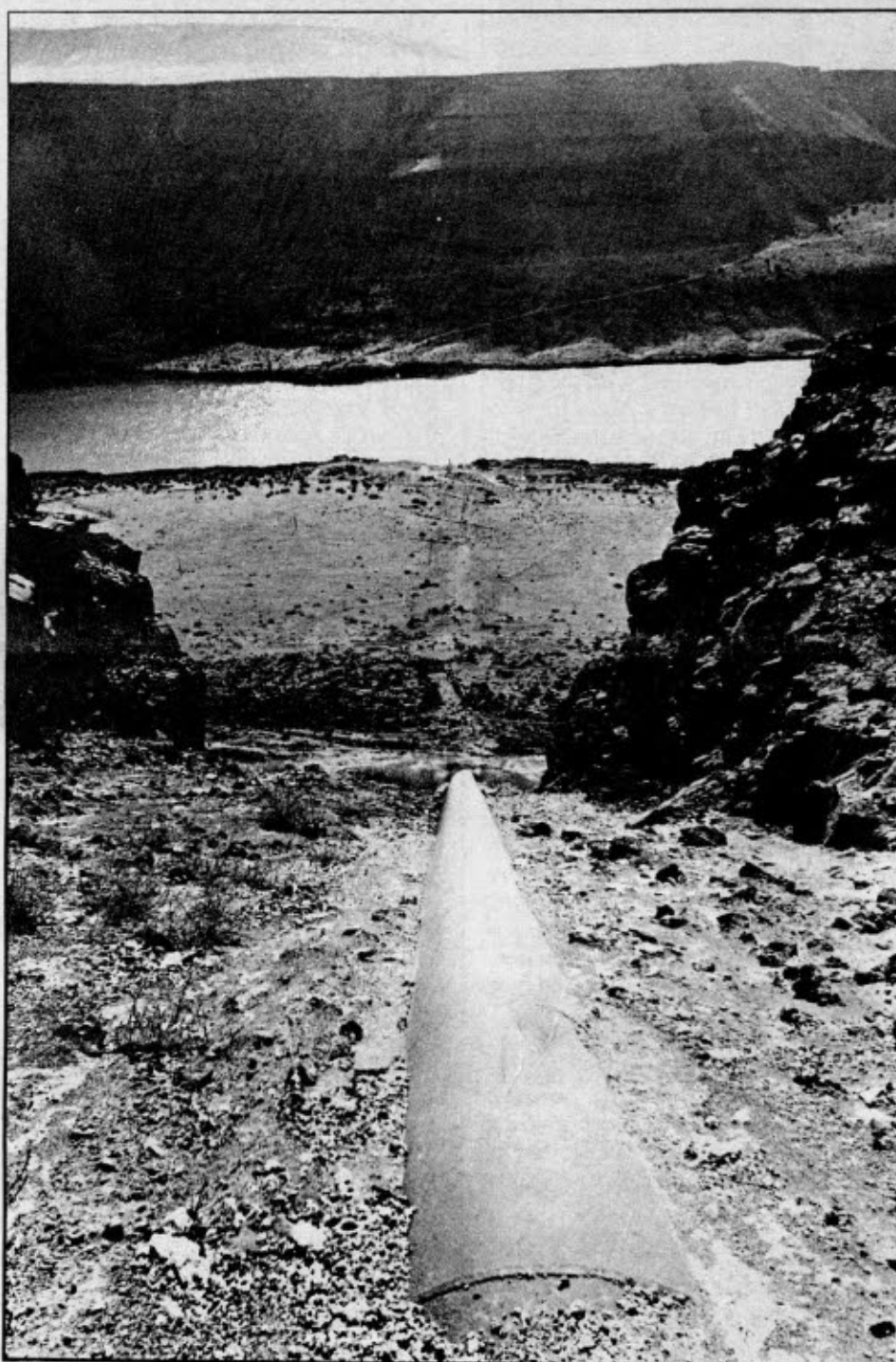
High lift pipeline conveys irrigation water from Snake River canyon
