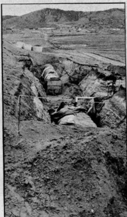
Foothills Water Treatment Plant under construction
