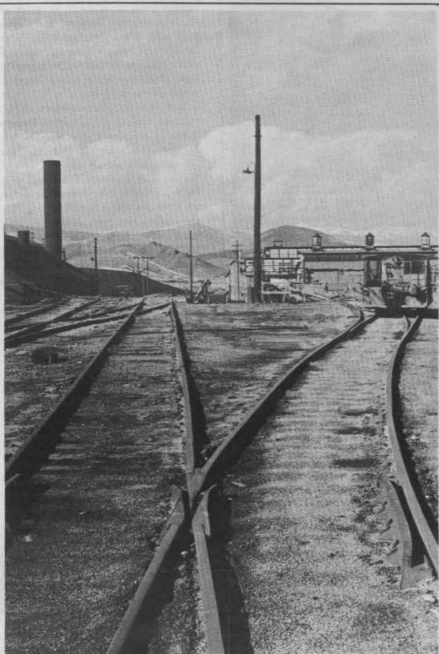
RAILROAD TRACKS at the copper smelter in Anaconda, Mont., lie unused and await the wrecker's bar.
