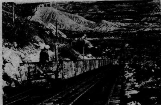
Utah State Historical Society photo THE TRAMWAY AT HIAWATHA, around 1940. Loaded cars were lowered by cable to the cleaning plant two miles below the mine mouth. Today the tram stands idle, despite the new boom in Utah's coal fields.
