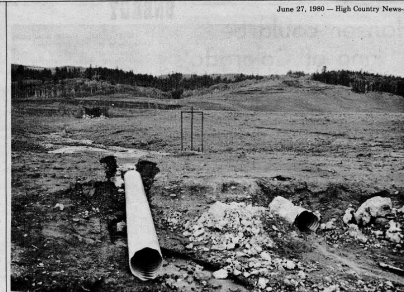
SOMETIME LAST WINTER, this Alunet check dam, along with the larger holding pond dam in the background, breached. Above the road cut is Alunet's open-pit phosphate mine. Alunet wants to open a much larger operation on Diamond Creek ten miles to the south.
