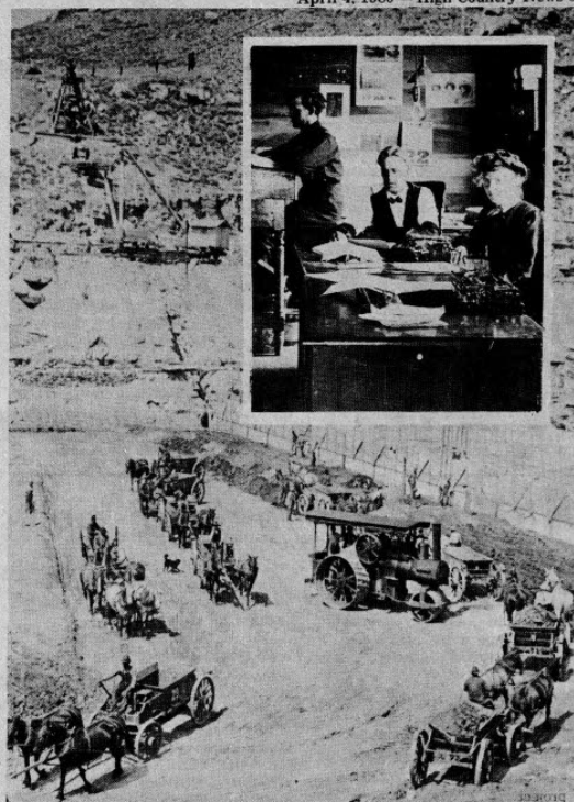
Photo courtesy of the Water and Power Resources Service
