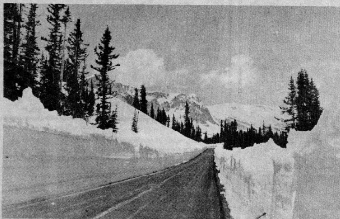
Wyoming Highway Department photo
