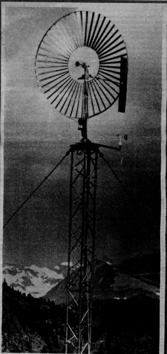
WIND slips down through a notch in the mountains at Eldorado Canyon to give the wind generators at Rocky Flats a stiff test. Shown here is one of the 16 machines at the test site, an American Wind Turbine.
