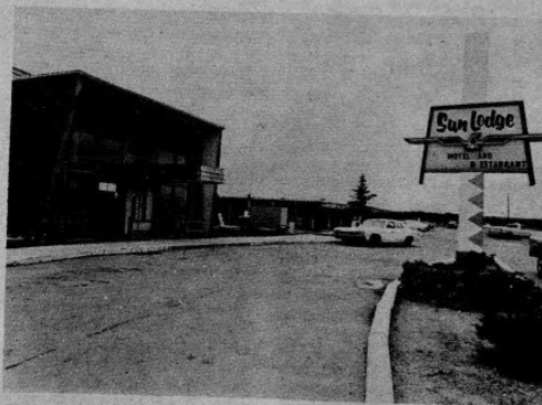
TRIBAL ENTERPRISE. Within the next 10 years, tribes will be outlining their future needs for water, for industrial, agricultural, and domestic uses as well as commercial enterprises such as this motel and restaurant on the Crow Reservation in Montana.
