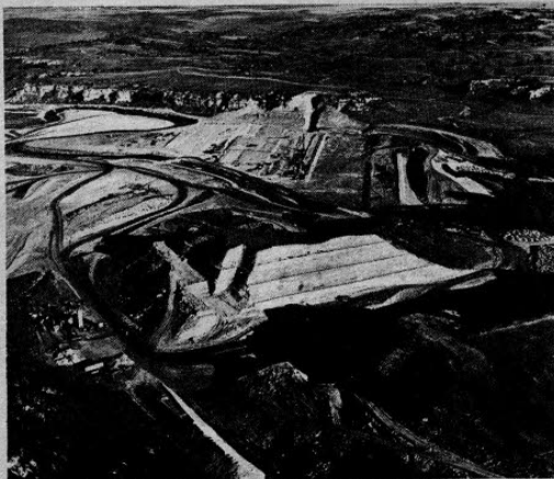
Photo courtesy of Tri-State Generation GRAYROCKS DAM and reservoir were about 25 percent complete when the judge issued his injunction to stop construction. Plaintiffs have now agreed not to erect further legal barriers to its completion.
